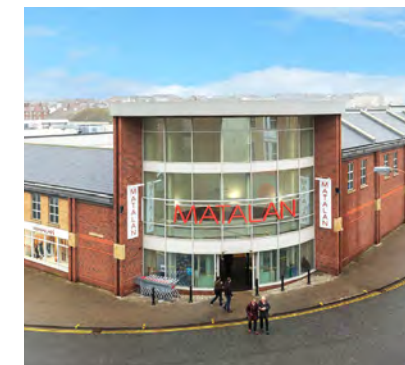
Matalan, St Thomas Street, Scarborough YO11 Modern purpose-built retail unit constructed in 2005. Let for 14 years to Matalan. Acquired for private overseas clients.
