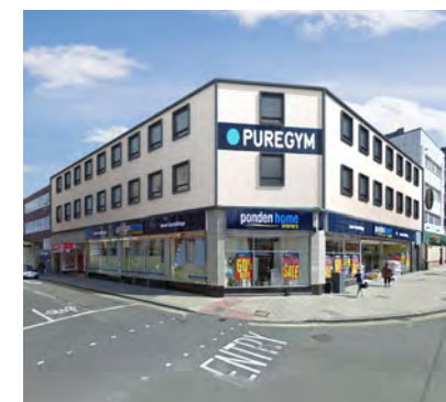
GYM PureGym, Croydon CR1 New leisure investment let for 15 years to PureGym with RPI rent reviews. Sold to a private investor on behalf of a developer.
