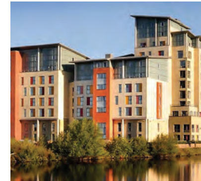
STUDENT Stockton on Tees TS18 Student block comprising 382-bed spaces. Acquired on behalf of an overseas investment fund.
