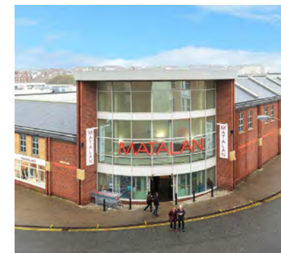
Matalan, St Thomas Street, Scarborough YO11 Modern purpose-built retail unit constructed in 2005. Let for 14 years to Matalan. Acquired for private overseas clients.
