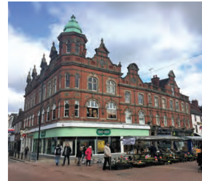
High Street, Burton-upon-Trent DE14 Freehold retail parade with residential upper parts. Sold on behalf of a UK family trust.
