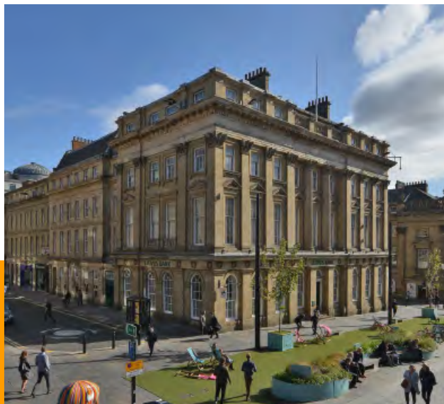
Lloyds Bank Plc, Grey Street, Newcastle-upon-Tyne NE99 Prime landmark city centre bank investment secured to Lloyds Bank Plc. Acquired on behalf of an overseas investor.
