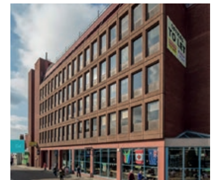
Brenchley House, Maidstone ME14 Substantial office and retail building with permitted development rights to convert to over 100 units. Acquired for a UK private client.
