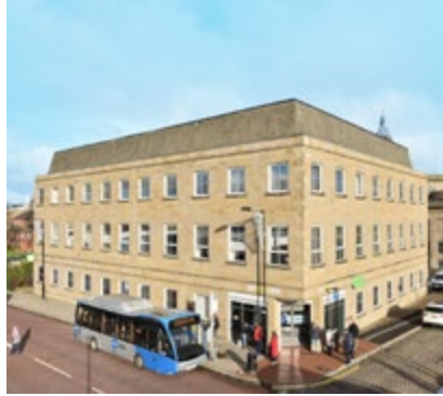
Black Horse Street, Bolton BL1 High yielding office building let to the Secretary of State. Acquired for a UK property company.
