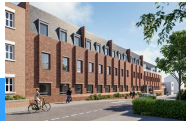
Foundry (Maxet House), Luton LU1
