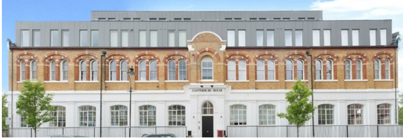
Canterbury House, Canterbury Road, London NW6
