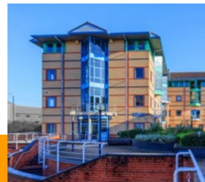
Bridge House, Dudley DY Modern office building close to the Merry Hill Shopping Centre. Acquired for a UK property company client.
