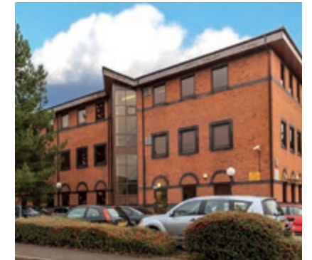
Barclays House, Cardiff CF14 High yielding office building let to Barclays bank. Bought and sold on behalf of a private client.
