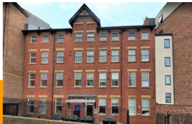
Albion House, Newcastle NE1
