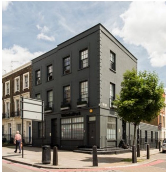
Camden Road, London NW1
