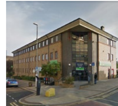
Shildon House, Gateshead NE8 High yielding office building let to the Secretary of State. Acquired for a UK property company.
